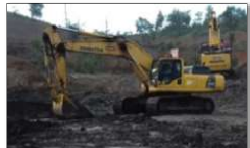
Gambar 4.3 Excavator Komatsu PC 400
