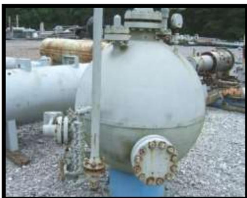
**Gambar 2.9. Separator Spherical**
